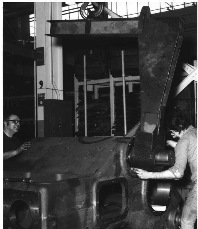
FIGURE 12 – JACKSHAFT REMOVAL/INSTALLATION FIXTURE
